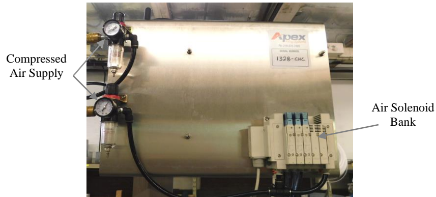
Figure 5-3 Air Solenoids
